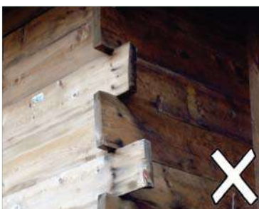
Boards ends not protected, nailed at weak location.
