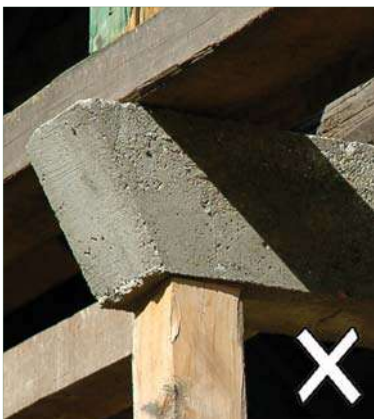
RCC beam has no connection to the timber posts. The frame is not well connected. Framing must be all timber
