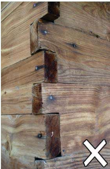
Boards ends not protected, nailed at weak location.
