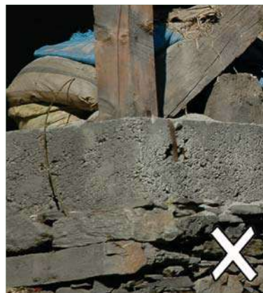
RCC beam has no connection to the timber posts. The frame is not well connected. Framing must be all timber
