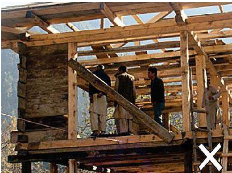
Distance from the corner to opening must be minimum 5 ft.
