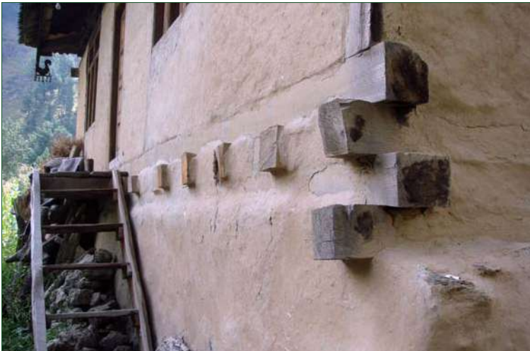
A good plinth protects the base plate and ensures it dries quickly.
