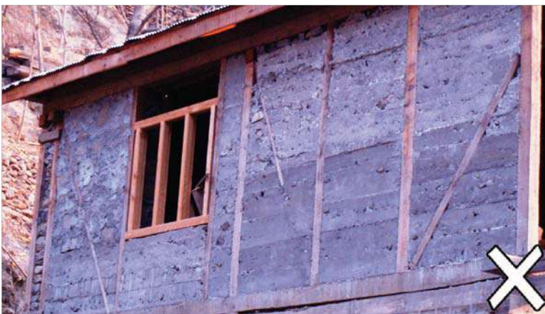
In situ concrete infill.
